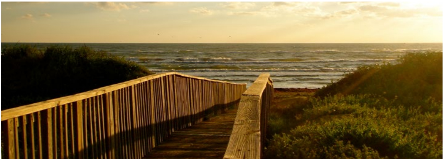
Example of a beach access point over a dune on South Padre Island
